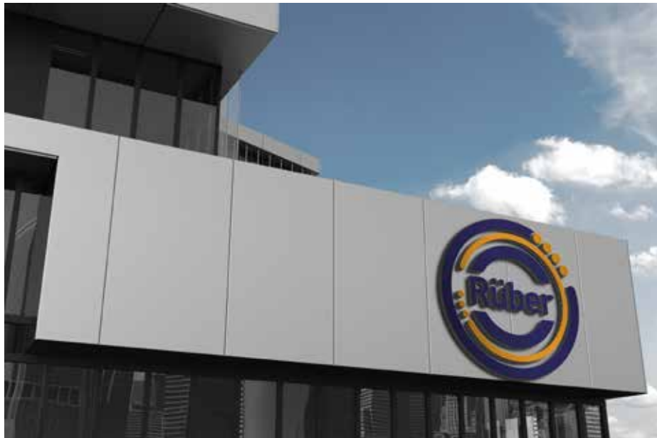
Rüber Headquarters - Bogotá Colombia
